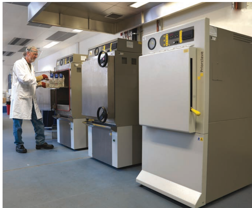
This multiple autoclave installation carried out by Priorclave is indicative of the around-space required for service, with clear access to pipework.
