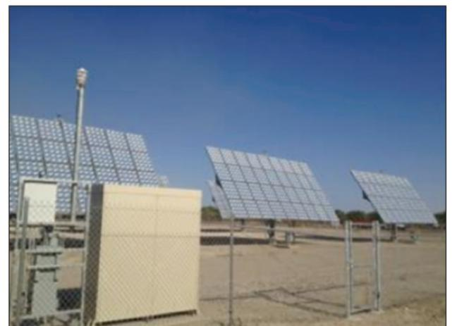
PV Monitoring: Lufft weather station W5501 in use on a PV farm in California, USA
