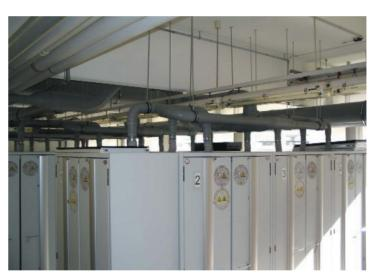
More than 50 safety storage cabinets connected to a central ventilation system
