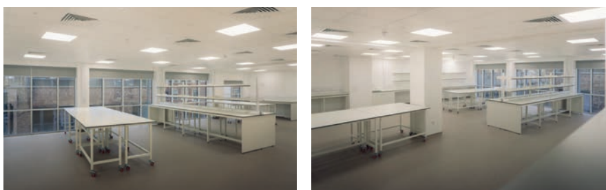
Laboratories fitted out in 85 Grays Inn Road for Clearbell. Credit Kastner Laboratory Design
